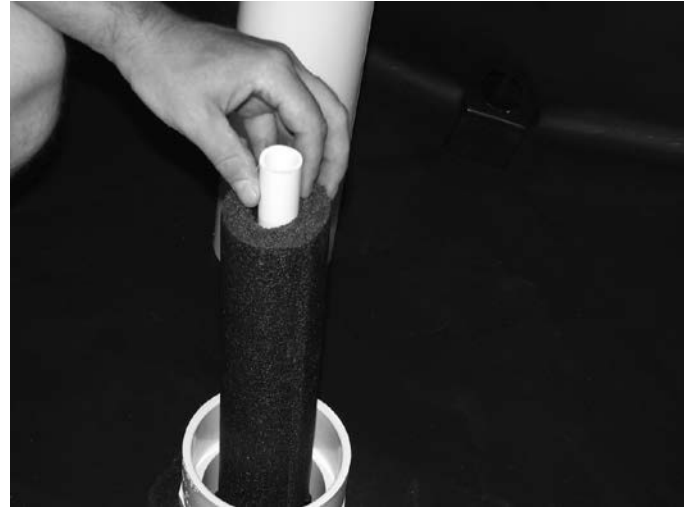
Step 8 Slide the pipe insulation on the \frac{3}{4} " (.95cm) fill line. Leave it about 1 \frac{1}{2} " (3.81cm) down from the top of the pipe.
