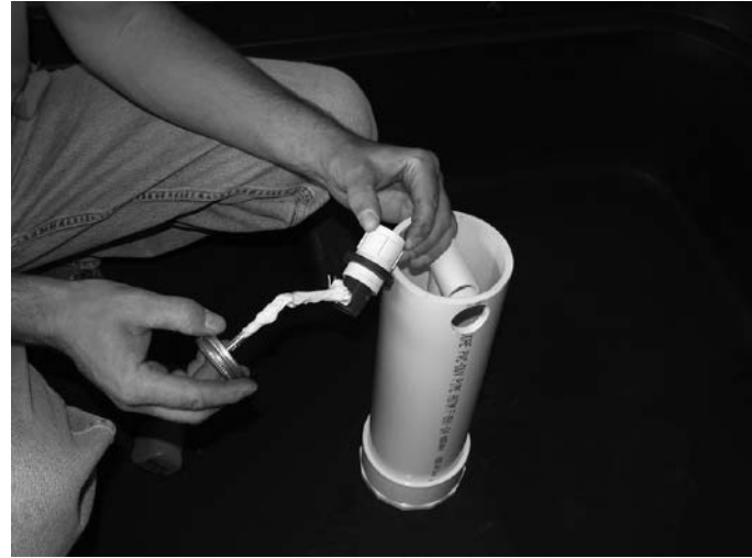
Step 14 Apply pipe dope to the 3/4" (1.90cm) pvc adapters.
