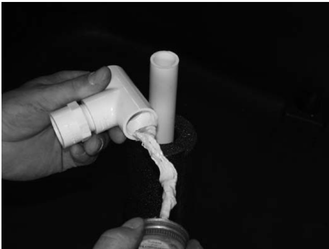
Step 9 Apply pipe dope to the threads of your fittings and screw it into place securely.
