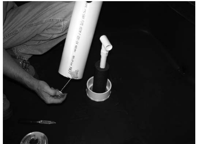
Step 12 Apply PVC cement to the bottom of your 4" (10.16cm) pipe.
