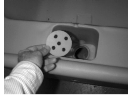
Step 9 Insert the poly drain screen in the overflow hole to keep unwanted debris out of the system for constant flow only, otherwise place a 3" (7.62cm) rubber drain plug in this opening.
